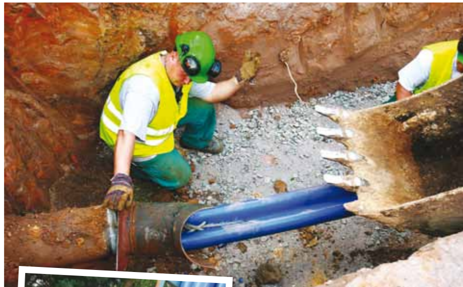
Above: The compact pipe is guided into the mouth of the old asbestos cement (AC) water pipe. Left: The Netherlands Ambassador to South Africa Rob de Vos broke a shovel to launch the Trenchless Technology pilot program.
