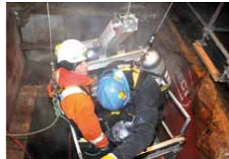
Temporary elevator for sewer access.
