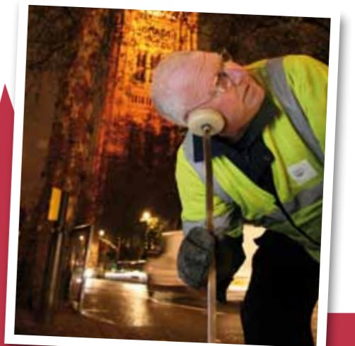
Checking for underground leaks outside Parliament.
