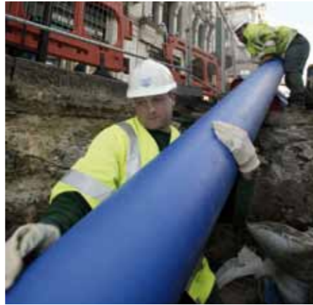
Renewing London's Victorian water mains Leicester Square.
