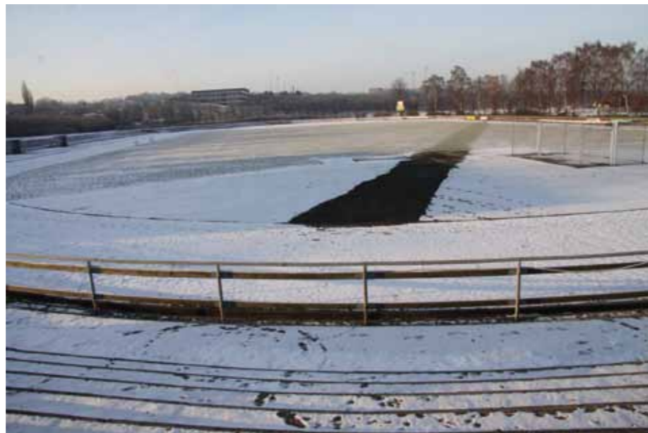
The pipe course below the playing field prior to renewal.
