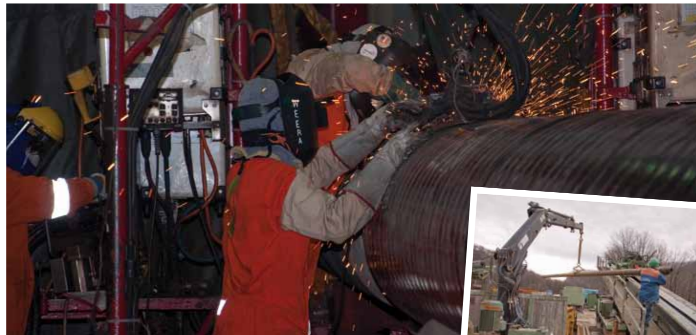
Manoeuvring pipe into place.
