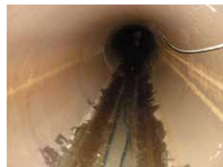
View of the face of the steel pipe DN 1,400 mm jacking.
