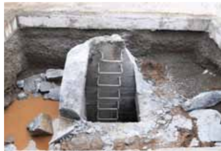
Manhole modification.
